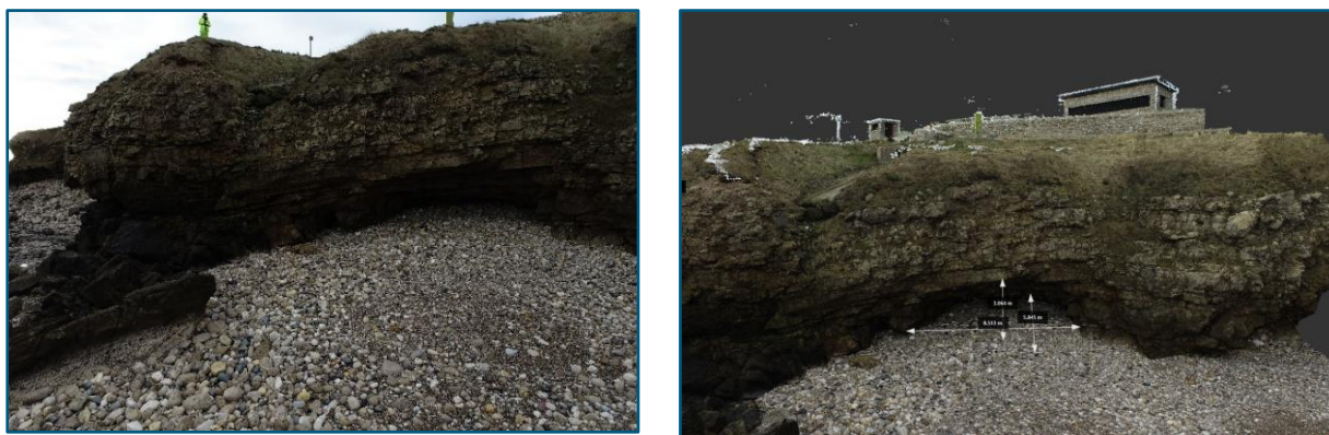
Cave 7 (Out of Study Area) - Approximately 8.5m wide, 3m high, 6m deep. (Left) Image from drone survey (Right) Annotated RGB point cloud
