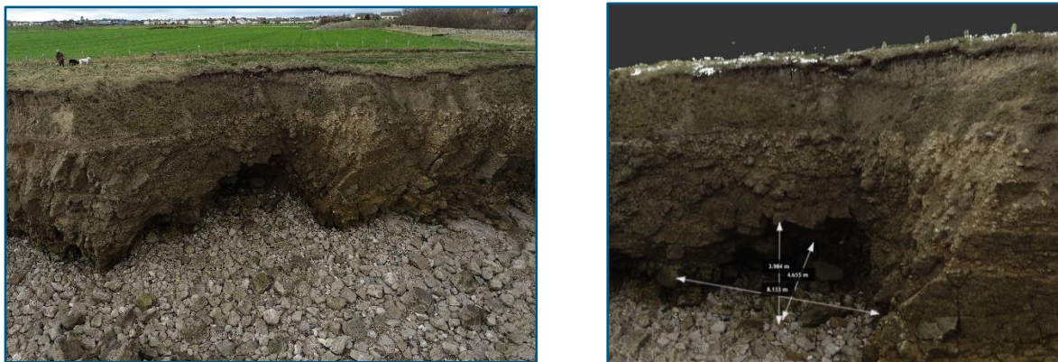
Cave 6 (Area F) - Approximately 8m wide, 4m high and 4.5m deep (Left) Image from drone survey (Right) Annotated RGB point cloud
